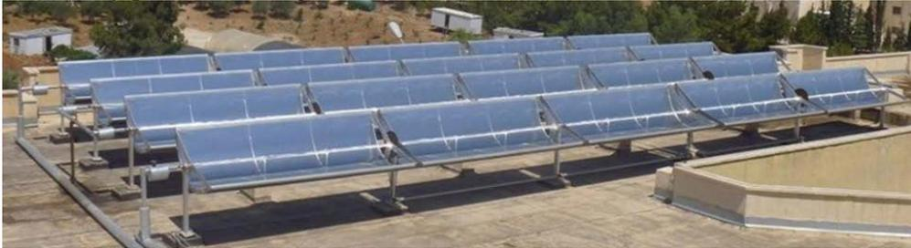
**Figure (1) Parabolic Trough Collectors**
