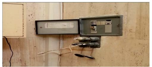
Figure- 17(c): Exposed electrical box in KCBB.
