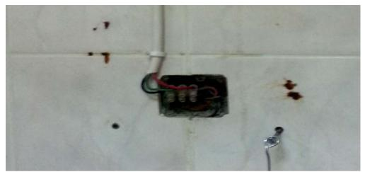
Figure- 17(a): Improper electrical output source.
