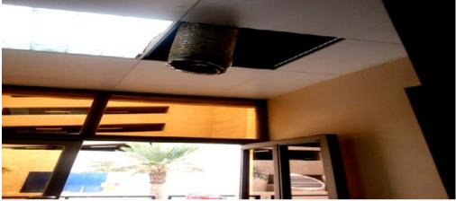
Figure- 16(a): Broken air conditioner.
