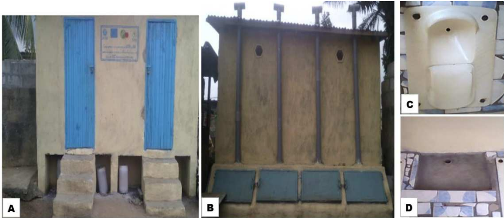
Figure 1. Dry composting toilets monitored in the experiment. A. Front view; B. Rear view; C. Orifice for urine collection and valve covering the pit; D. Wastewater collecting orifice (wastewaters are from hand and anal washing water after each defecation).
