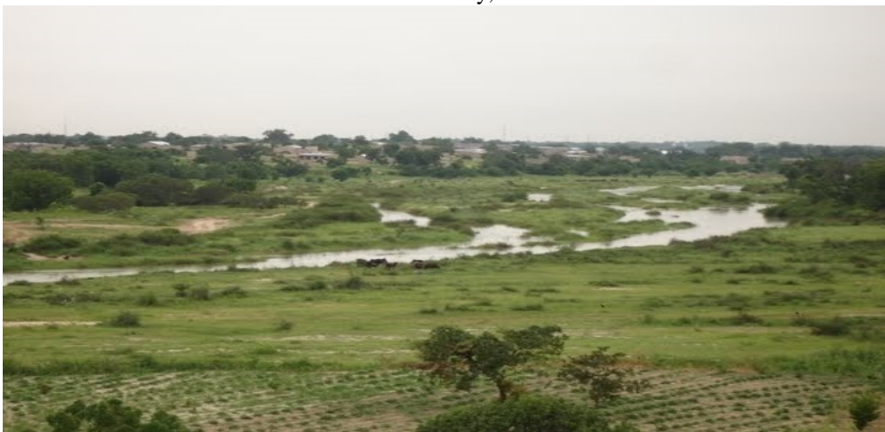
PLATE 5: THREAT TO FARMLANDS DUE TO CONSTRUCTION OF ALAU DAM (SURVEY, 2013).
