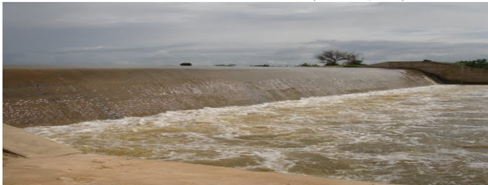
PLATE 2: ALAU DAM OVER FLOW CHAMBER (SURVEY, 2013)
