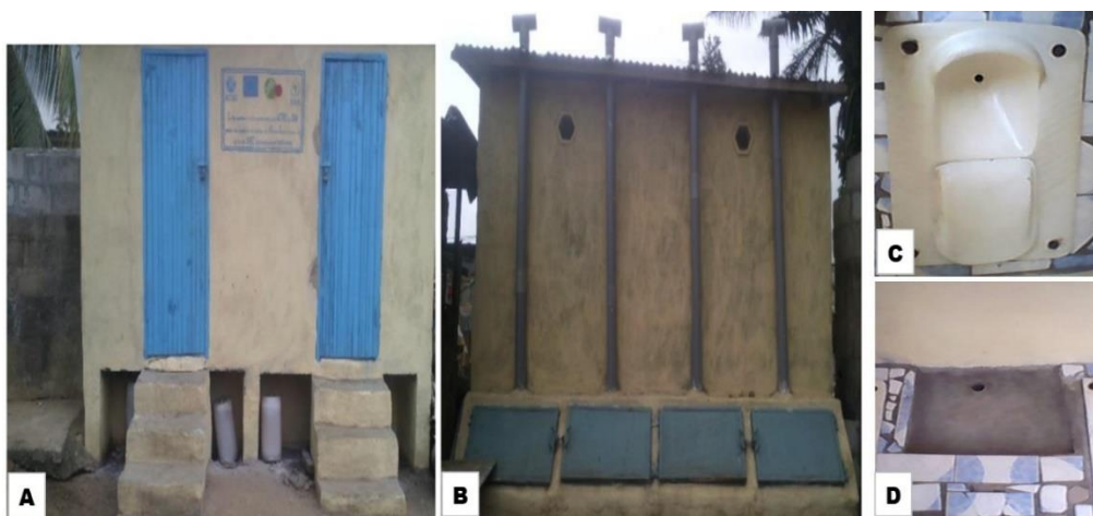
Figure 1. Composting toilets monitored in the experiment. A. Front view; B. Rear view; C. Orifice for urine collection and valve covering the pit; D. Wastewater collecting orifice (wastewaters are from hand and anal washing water after each defecation), (Effebi et al., 2017)
