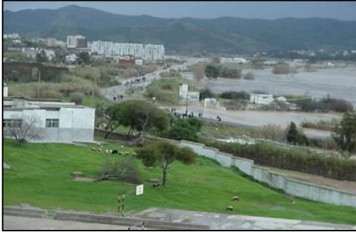
Figure 2: Flood of Tetuan city: area between Romana and the bus station (Hotel Pristigia now).
