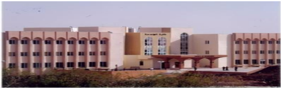
Figure-8 Building of Engineering Faculty
