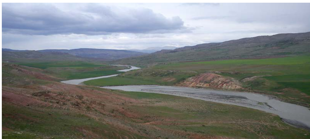
Fig 3. Kezer regulator and HEP route of the transmission channel
