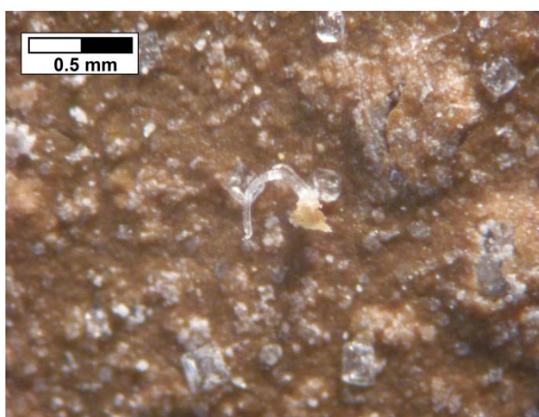
Figure 6 – Needlelike efflorescence causing spalling.
