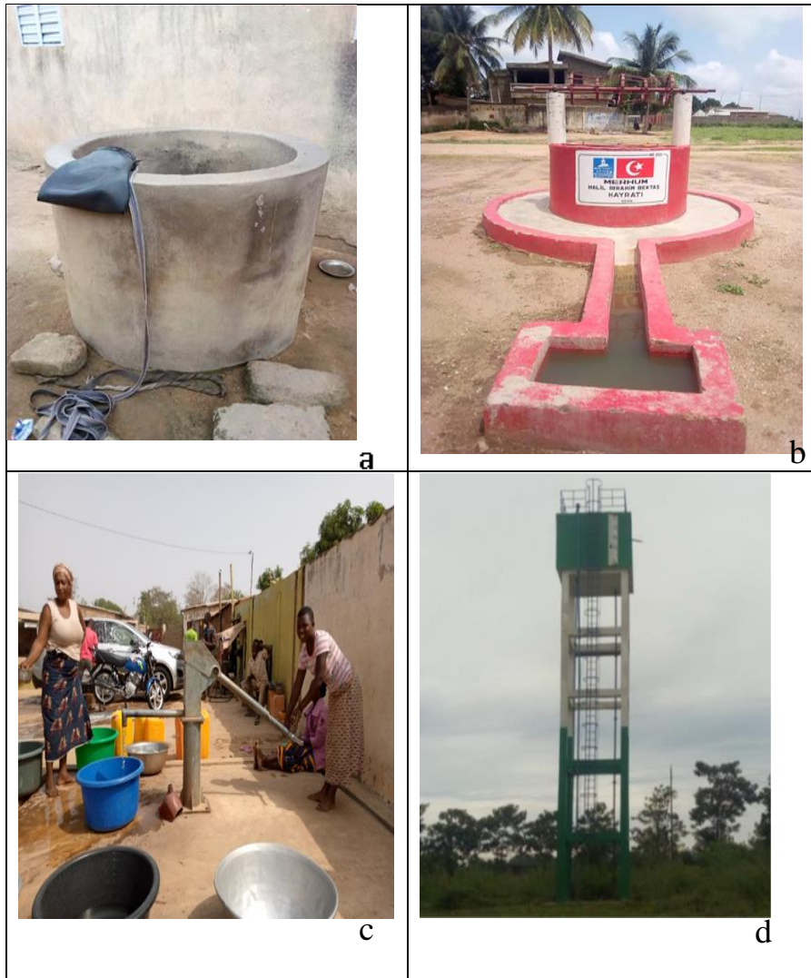
Plate 1: Hydraulic infrastructures of the city, a: traditional well; b: modern well; c: manual drilling; d: an autonomous water station.
