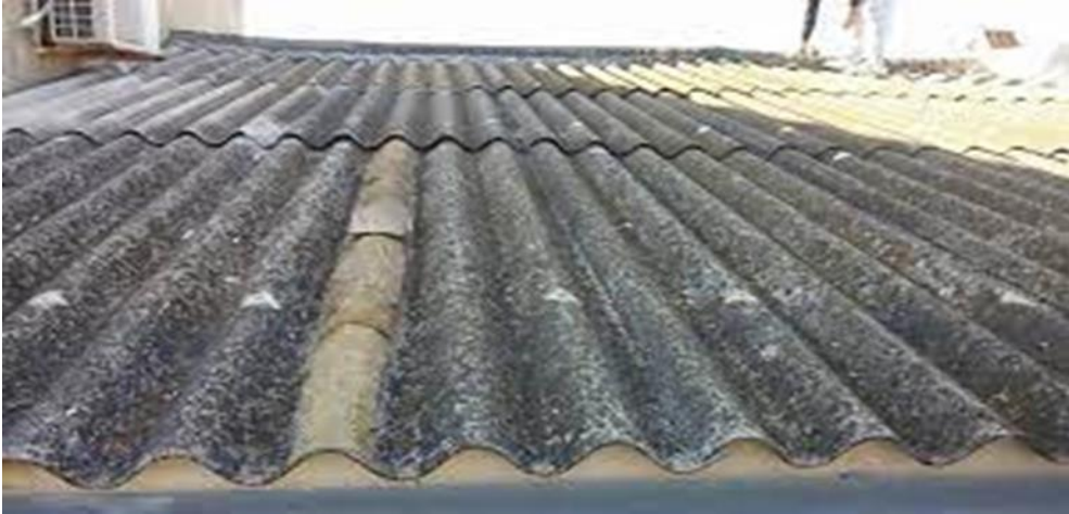
Figure 1: Asbestos asbestos sheet used as a roof or shed, with a corrugated shape imitating a tiled roof (Elenit)
