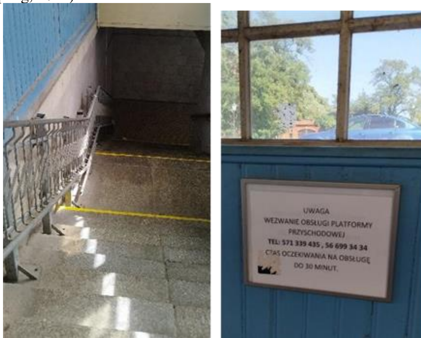
Figure 4: Examples of train stop infrastructure (stairs) and information not adapted to seniors needs. (phot. M.Bis)
