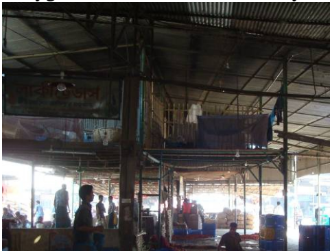
Figure 29: Existing accommodation system in drop slab in Jatrabari bazar
