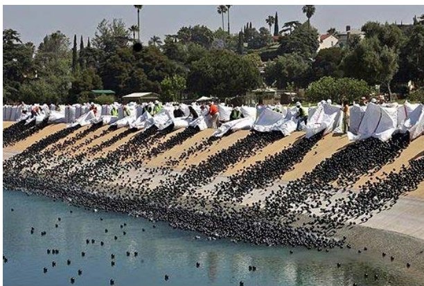
Fig.12: Black plastic balls on the water reservoir Ivanhoe on Silver Lake in Los Angeles (Source: http://www.trendite.net/2008/06/11/los-angeles-drops-400000-plastic-balls-into-ivanhoe-reservoir-to-block-carcinogen/ ).
