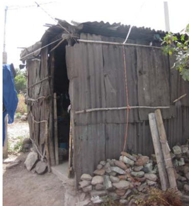
Fig. 3 House in Azumiatla built with cardboard, it has no windows.
