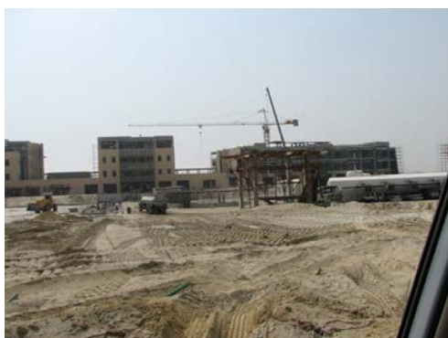
PMU-campus under construction, early 2007 © 2007 Profanter Annemarie
