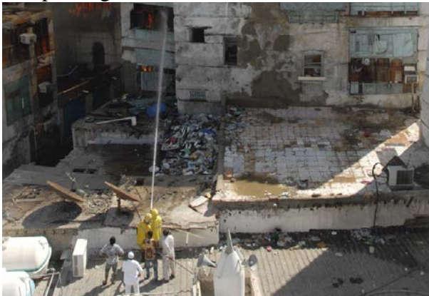
Fig.3. Collapse of buildings. (Week Online, Jun 30, 2010)
