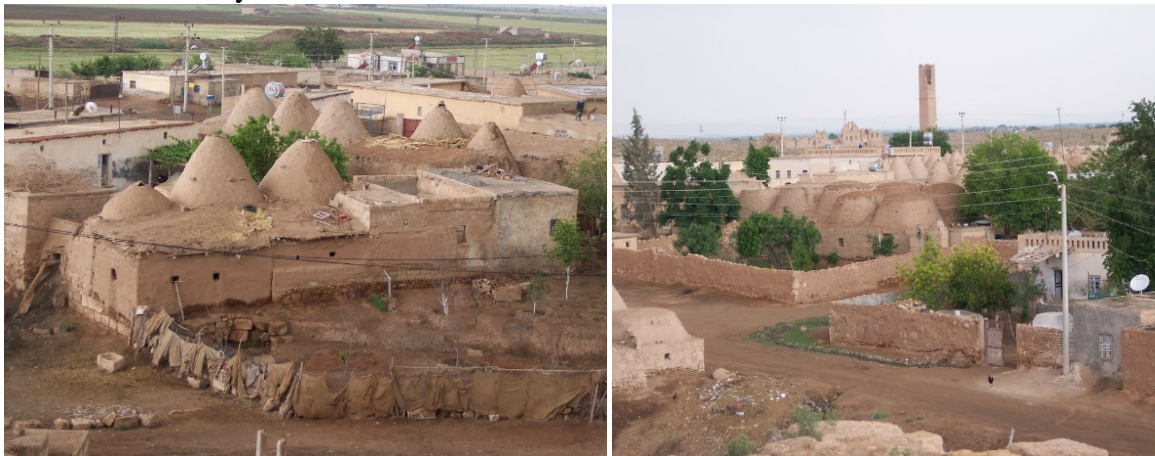
Picture 6. Conical shaped adobe structures in Akçakale (Ref. http://www.panoramio.com/photo_explorer#view=photo&position=5258&with_photo_id=74065596&order=date_desc&user=709943 )
