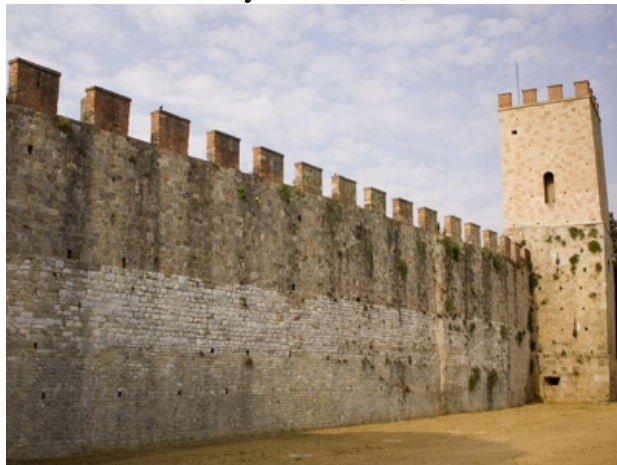
Source: ask.com .Old Roman City Wall and tower
