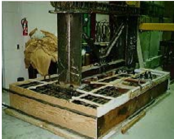
Fig.3: foundation framing and rebar placing and rebar placing of concrete slab
