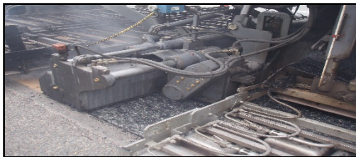
Figure- 6 Scarifying and heating unit
